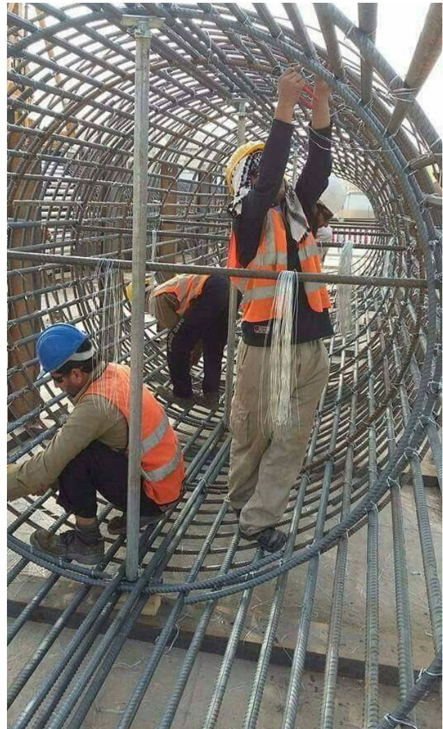
Workers on Lusail Stadium, where the Final of the FIFA World Cup Qatar 2022 will be played, described experiencing tension and exhaustion because of their working and living conditions. © Equidem 2022
